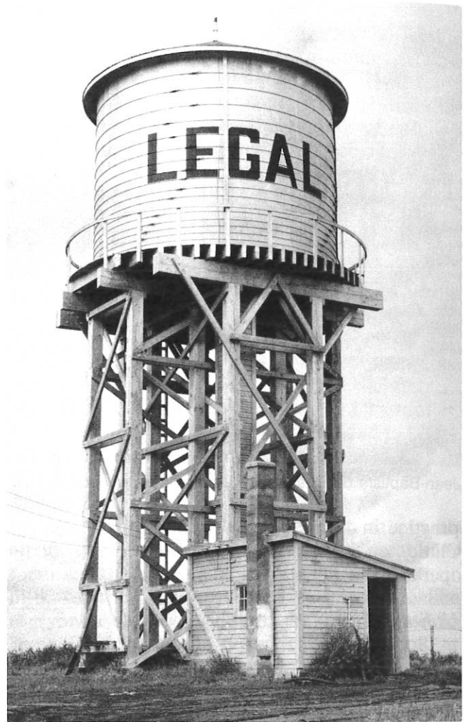
Legal landmark, 1963: the first reservoir with a capacity of 20,000 gallons of water was dug in 1958. A pumphouse was also constructed in order to pump water in a giant wooden tank sitting on top of a large wooden tower, situated on the west end of town, just north of main street
