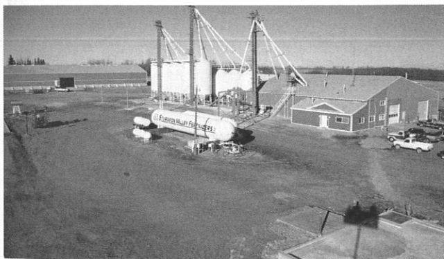
Sturgeon Valley Fertilizers Ltd., 1982, established in Legal with ammonia tank; 1986, built plant, 1986-93, three expansions built; 1994, new 70' x 270' 7000 MT bulk fertilizer storage warehouse. Future 40' x 40' heated chemical storage warehouse (lower right)
