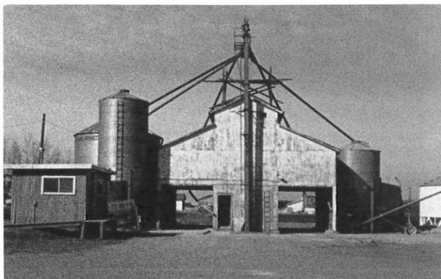
Seed-cleaning plant, built in 1959
