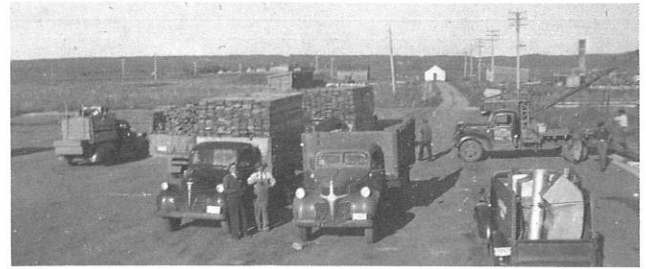
Loading trucks during the Penhold hangar demolition
