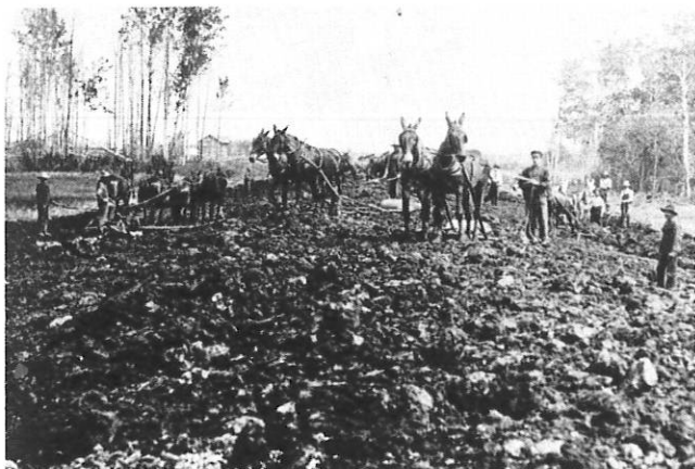
Construction of railroad between Morinville & Legal, en route to Athabasca; June 1909
