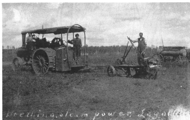
Introducing steam power. Logansville One of first steam engines in this district. Breaking land in the early 1920's are Emile Létourneau (at the wheel) and Eddie Létourneau (operating the plough-levers).
