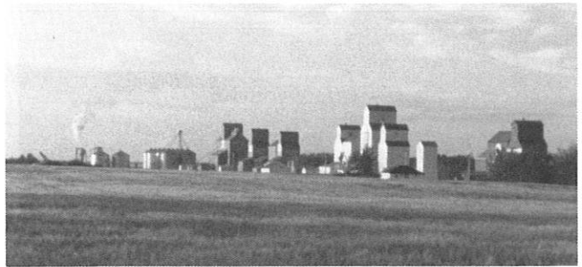
Legal Alfalfa Plant and Grain Elevators
