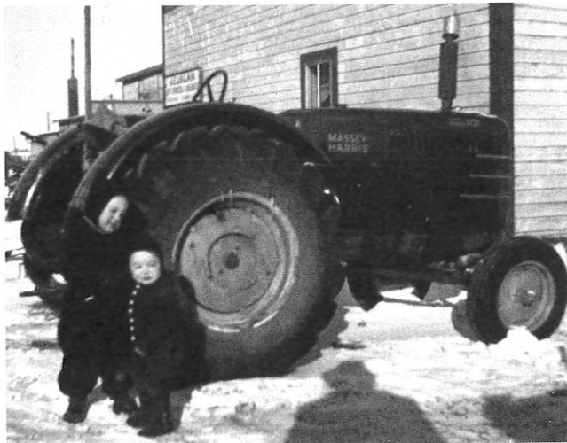
Laurent & Paul Cyr by Welding Shop & Massey Harris
